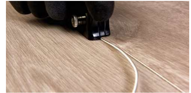
Figure 6.5 Cutting in the seams
