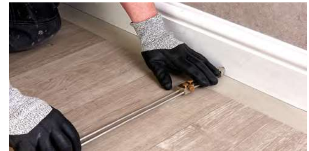
Figure 6.2 Scribing the wall profile
