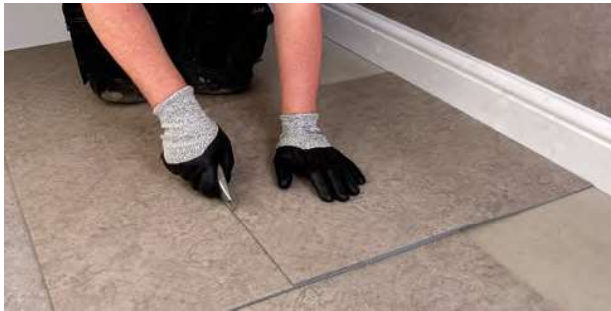
Figure 6.8 Measuring using an overlapping tile
