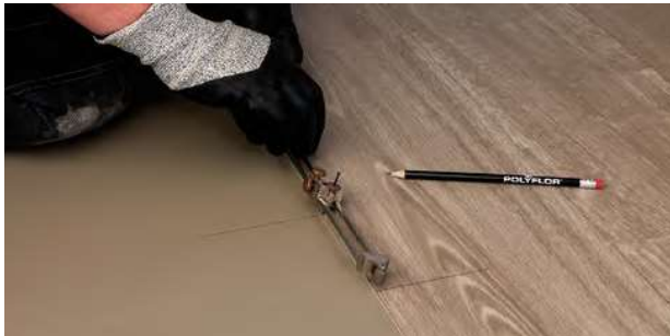
Figure 6.4 Scribing the wall profile
